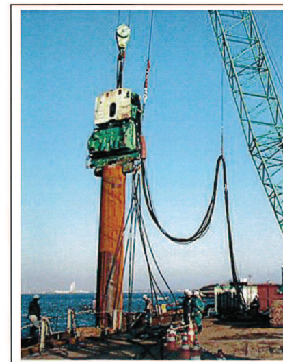
Piling, vibrating hammer
