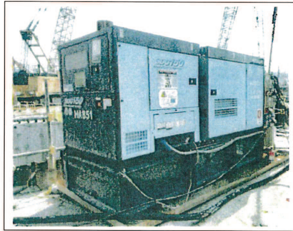
Generator, with Quality Powered Mechanical Equipment Label showing a Sound Power Level \leq 95\text{dB(A)}
